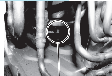
Nut of compressor fixing bolts
